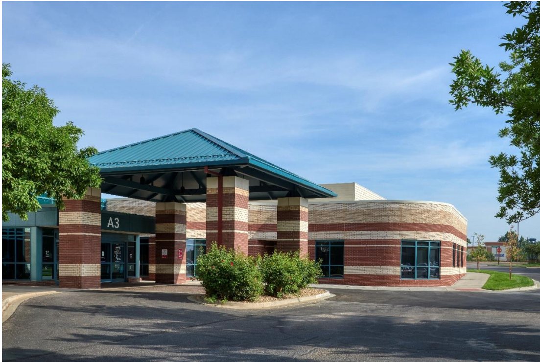
1: The main entrance to UCHealth Harmony Cancer Center with the new building addition on the right side of the photo.
