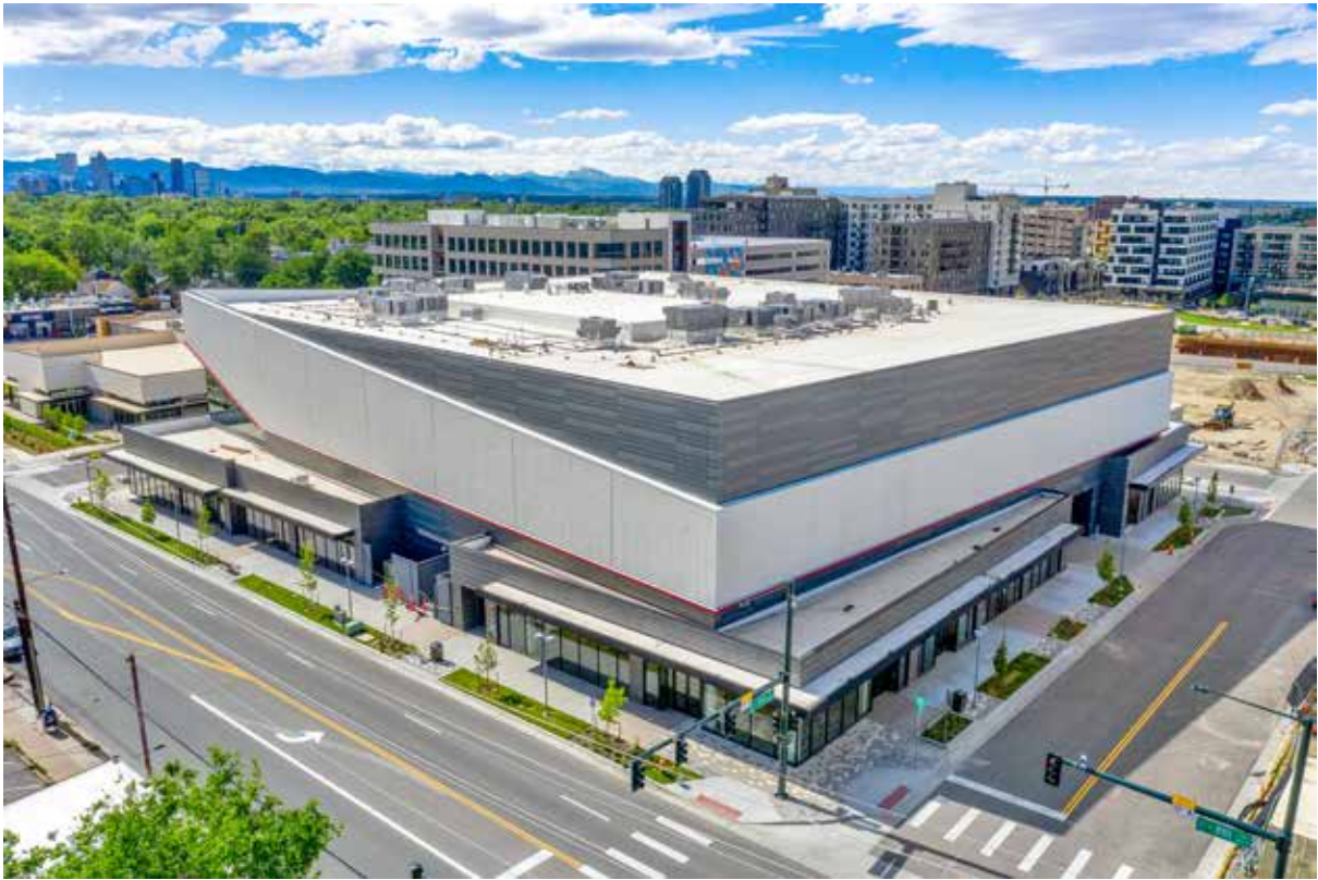
Birds-eye view of Block 2 shows northwest facing corner of the theater building with surrounding street level storefront for retail and restaurant. Photo by Kaarl Hoopes, Falcon Aerial Imaging.
