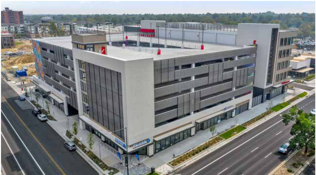
Northwest corner of Block 4 at the corner of 9th & Colorado. Birds-eye view shows multi-use building with office, parking and street level retail and restaurant. Photo by Kaarl Hoopes, Falcon Aerial Imaging.
