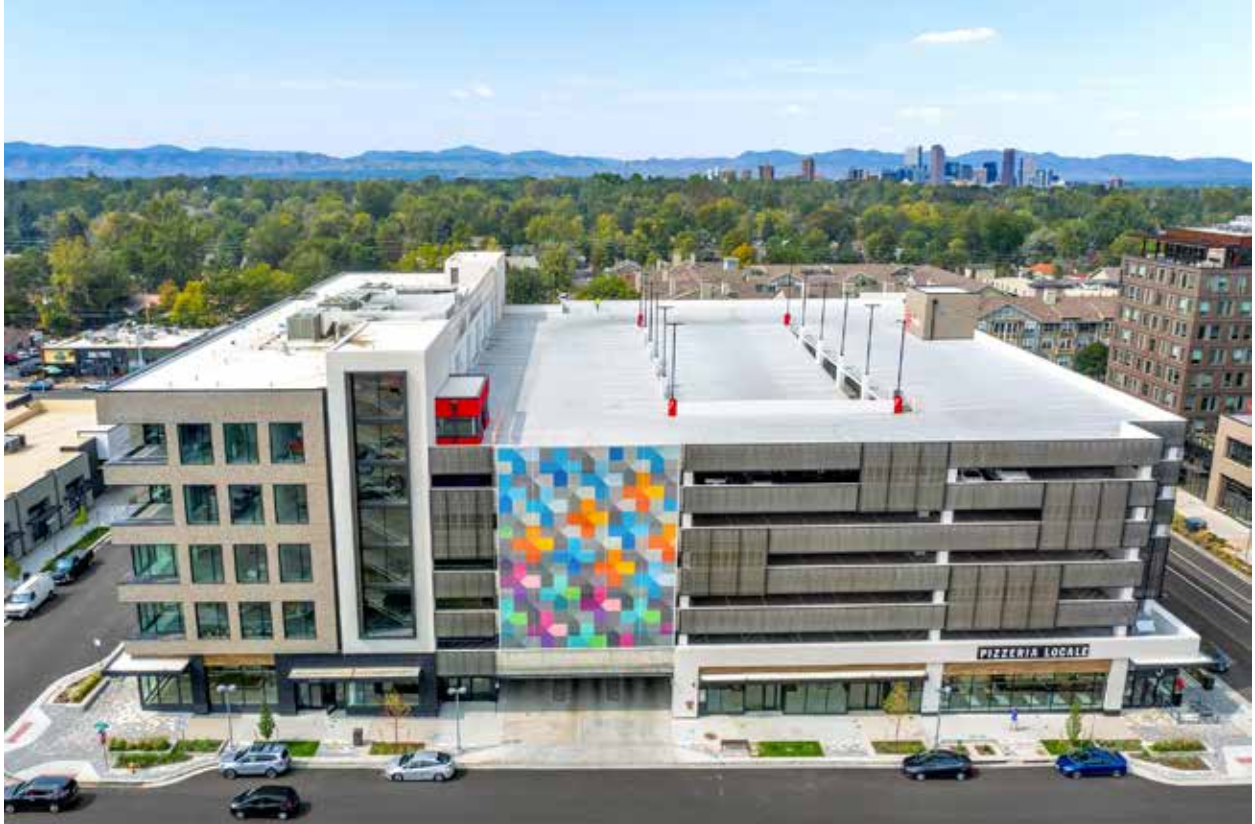
East side of Block 4 looking towards Denver. Birds-eye view shows the multi-use building with office, parking and street level retail and restaurant. Photo by Kaarl Hoopes, Falcon Aerial Imaging.
