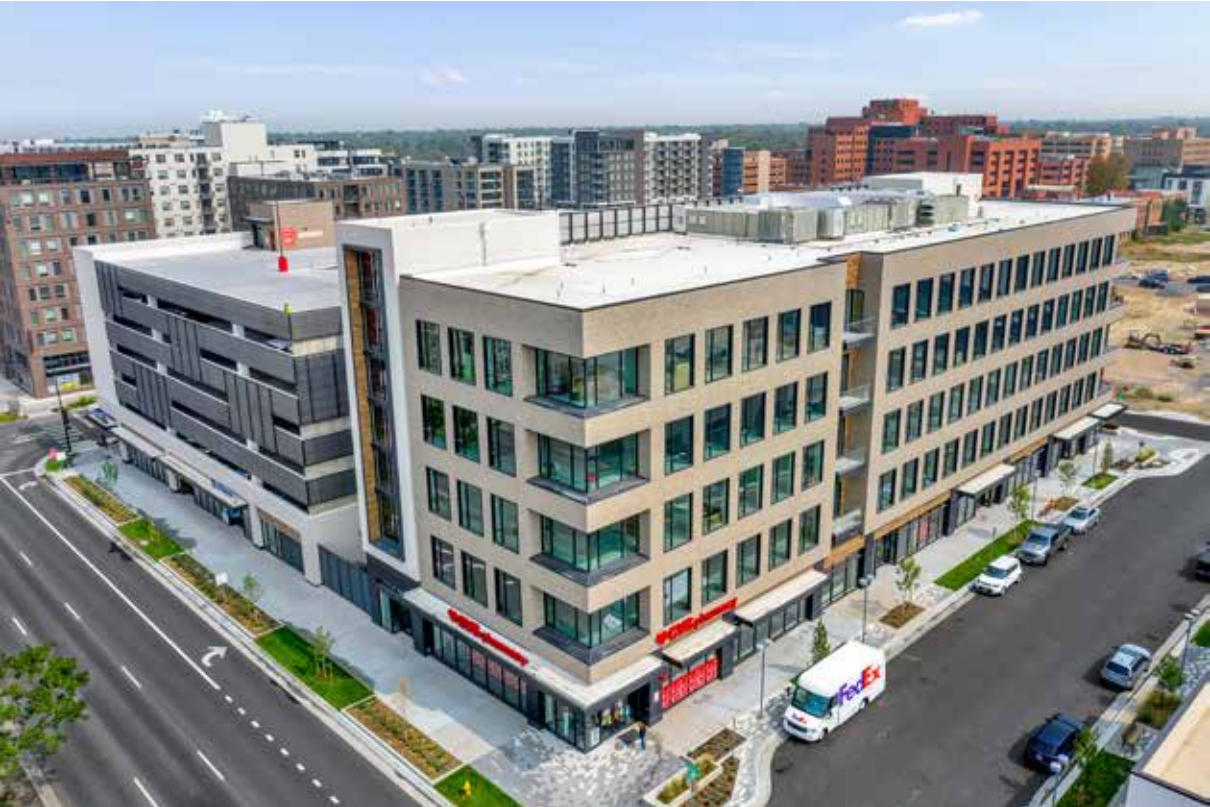
Southwest corner of Block 4 facing the multi-use building with office, parking and street level retail and restaurant. Photo by Kaarl Hoopes, Falcon Aerial Imaging.
