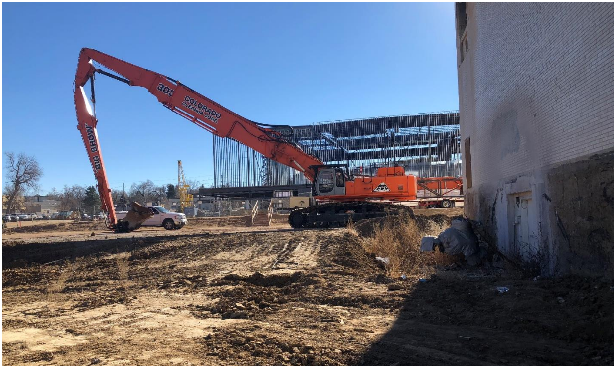
Photo 2: "The Big Show," CCC's High Reach Excavator
