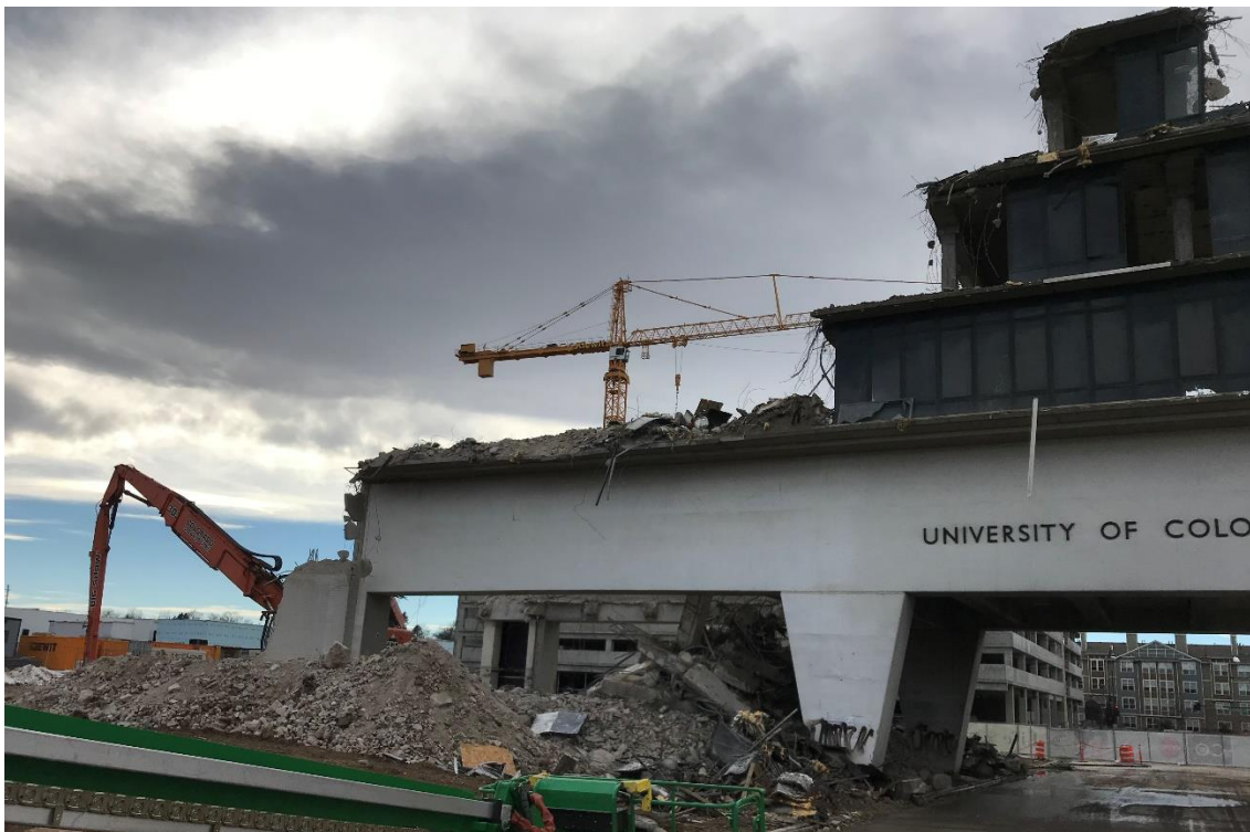
Photo 10: Demolition Begins on the Girder Sections
