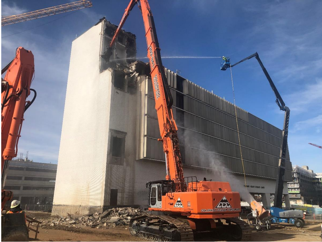
Photo 5: Dust Mitigation Techniques in Action
