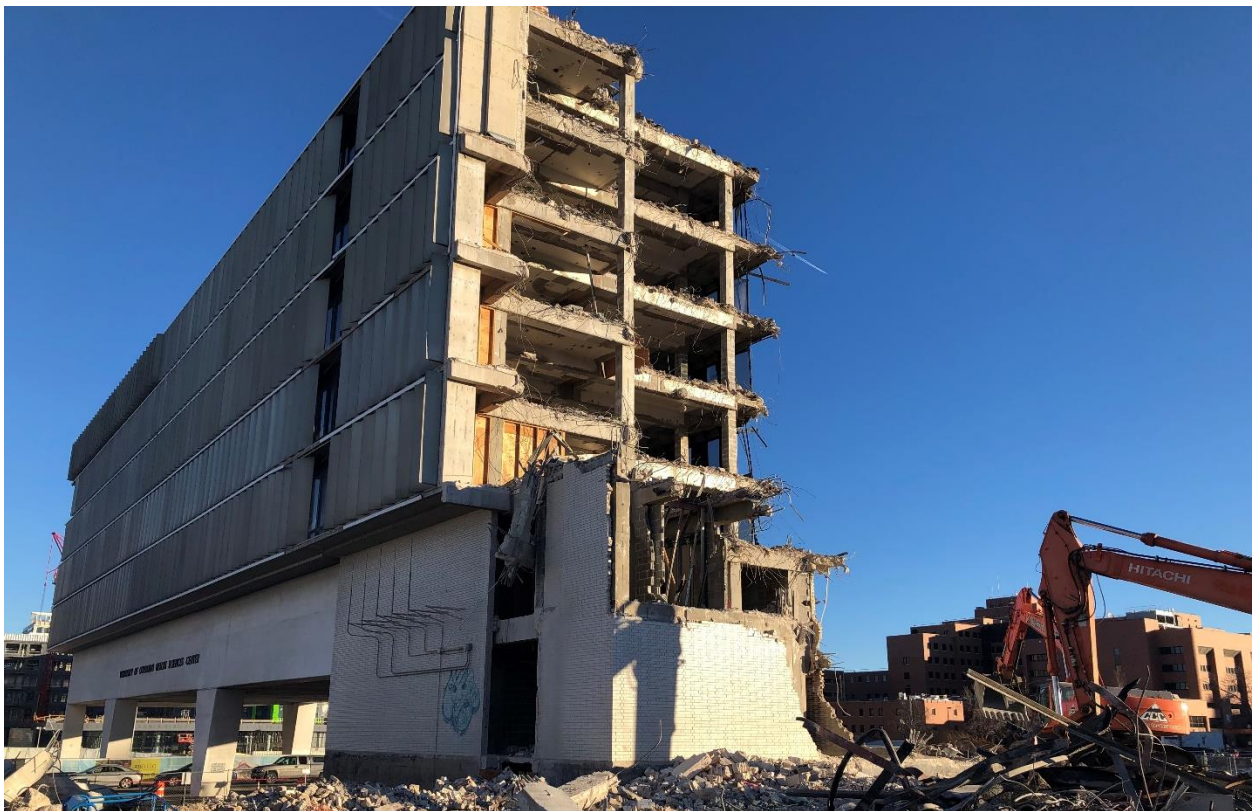
Photo 6: Building Cap on South End Nearly Completely Removed
