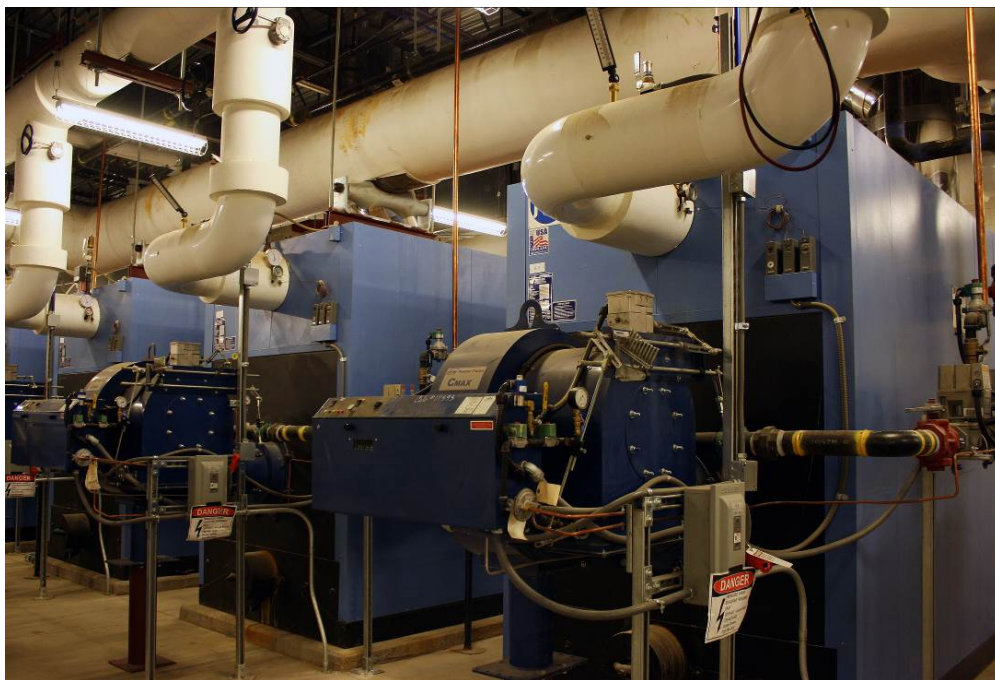
Boilers in Mechanical Room
