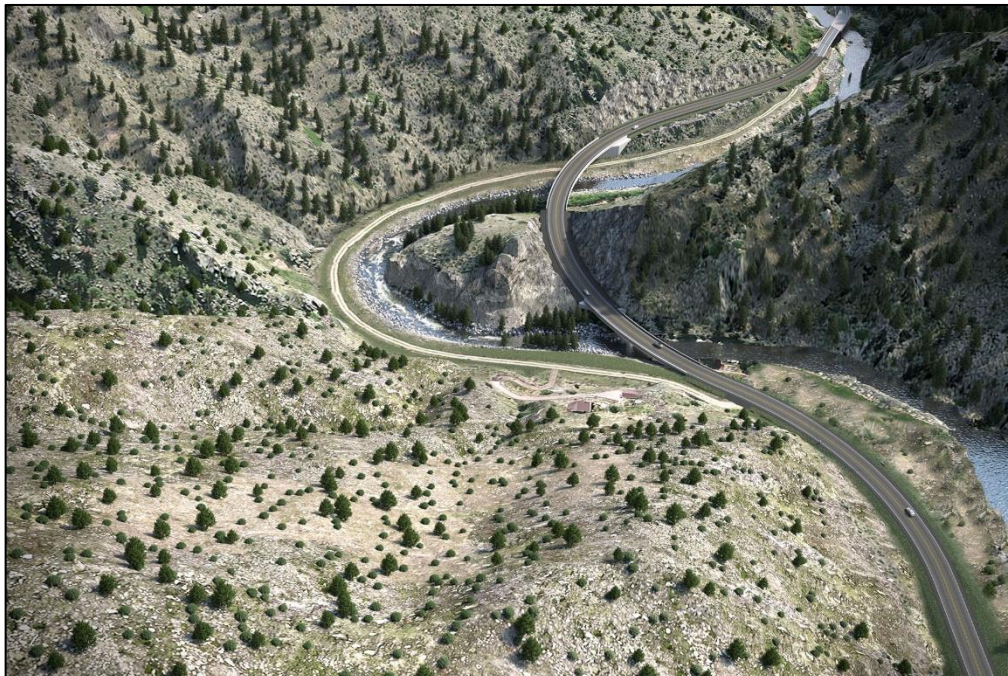
To help the public better understand the improvements being made through the "horseshoe curve" area of the inner canyon, the project team developed this rendering showing the realigned roadway above the river.
