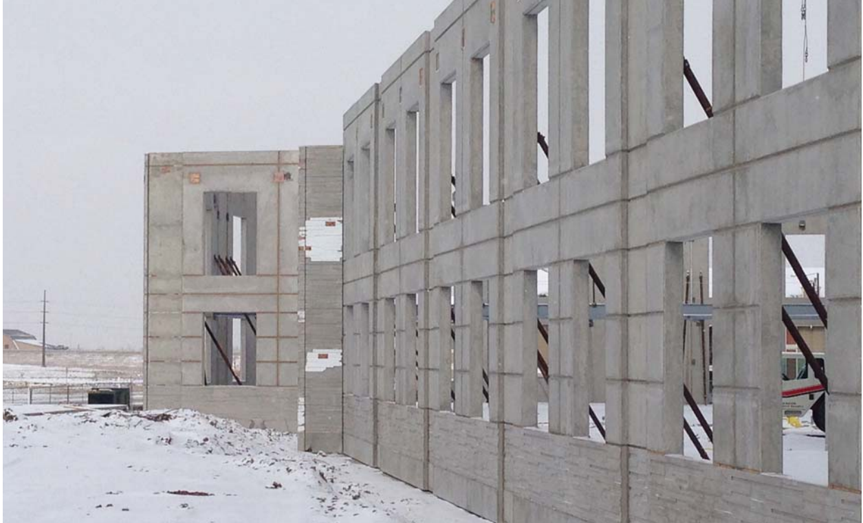
Tilt-up panel erection during winter months.
