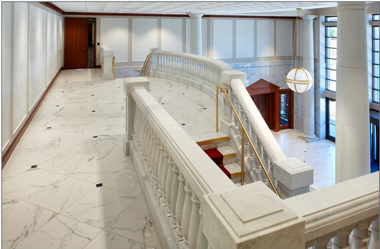
The first floor lobby showcases a dual grand staircase with hand-carved marble balusters and balustrades. Swinerton 3D scanned and modeled the balusters as each one sits directly on the structural steel framing to create the curved staircase to ensure accurate fabrication in China.
