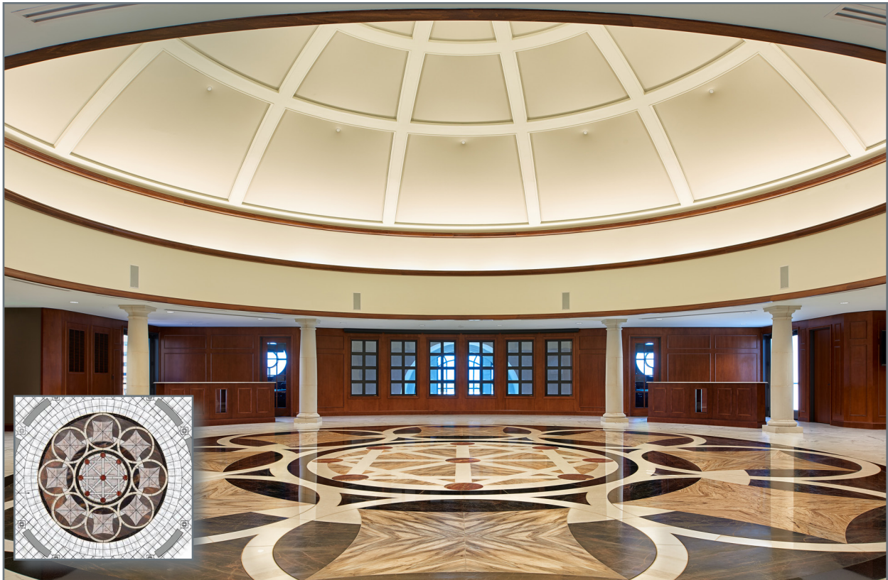
Over 4,000 pounds of pre-patinaed copper cover the dome. The lobby floor is covered by a 40-foot-wide stone medallion, and its design is based on the teachings of Greek philosopher Aristotle. The medallion installation took 2100 manhours, and the larger pieces weigh approximately 300 pounds.
